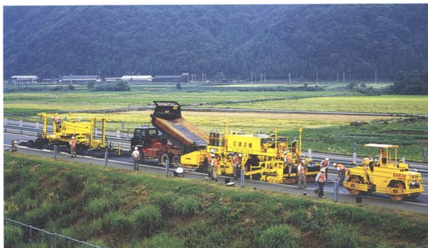
Re-Pave Hokuriku Expressway(1980s)
