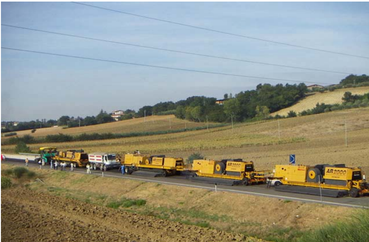
Figure 9. AR2000 under operation at site
